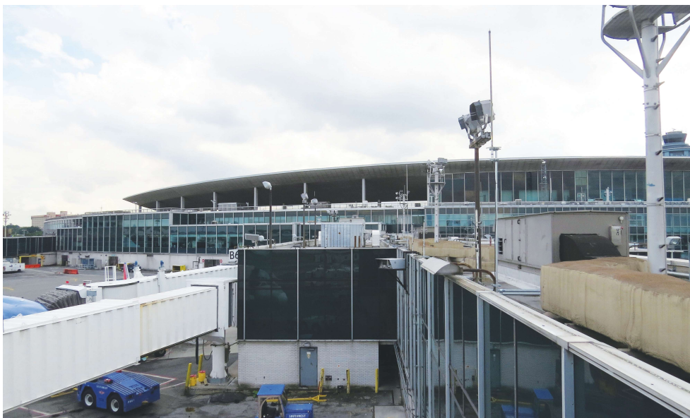
The Interceptor has several components but the sensor unit itself is small enough to fit on the top of an airfield antenna.
